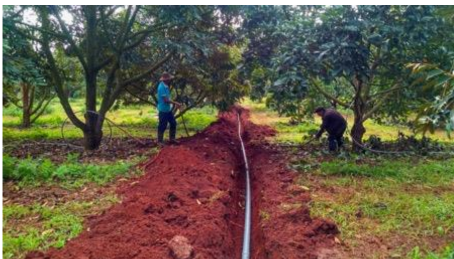
Figure 5. Image of installing a water-saving drip irrigation system to combat climate change for durian trees in Dak Lak
